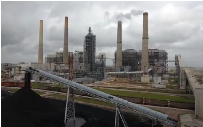
The Petra Nova 240 MWe carbon capture project at the WA Parish generating station, NRG Energy, southwest of Houston, Texas (JX Nippon Oil & Gas Exploration Corp., current owner)
